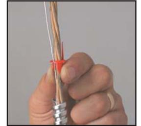
Insert the cable into the connector and secure the connector into the box. Be sure that the anti-short bushing is plainly visible in the connector for easy inspection. The same procedure is followed for traditional MC cable with the exception that there is no bonding wire. Although anti-short bushings are only required by the NEC® for AC cable, some manufacturers supply them for both cable types in the event that local codes override the NEC®.
